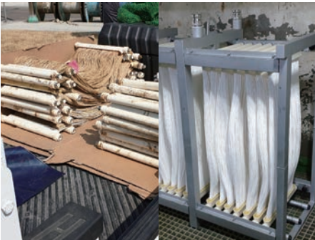
Replacement of membranes at wastewater treatment facilities
